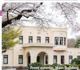
Front exterior, Main Building
