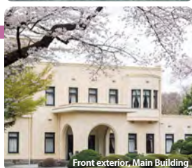
Front exterior, Main Building
