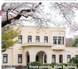
Front exterior, Main Building
