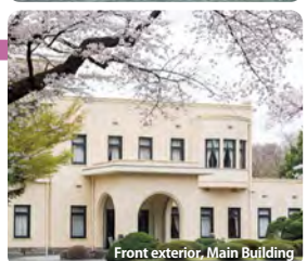
Front exterior, Main Building
