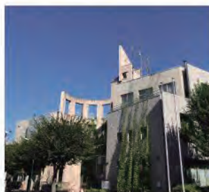
Itabashi Ecopolis Center
