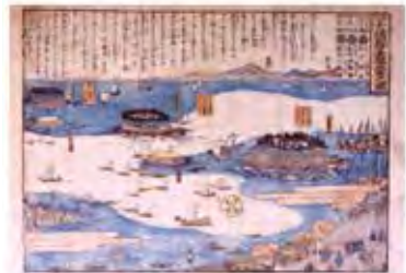
View of Odaiba's construction site as the Shinagawa artillery
