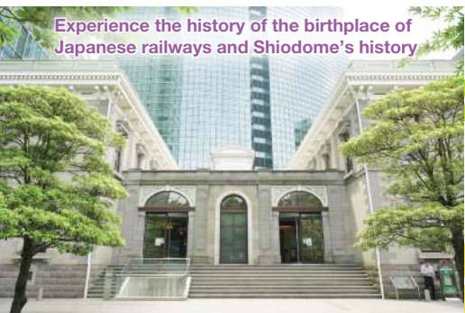
📍 The Shimbashi-Teishajo station building has been rebuilt in the same location as when it first opened
