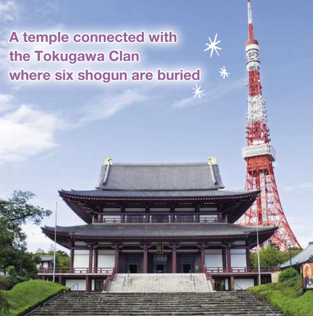
📍 Daiden, the largest temple hall in Tokyo *Under construction until October 2021. Open to visitors
